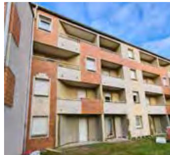
Coating on insulations
