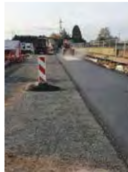
Realization of a bituminous base layer
