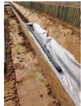
Installation of a rainwater drainage drain
