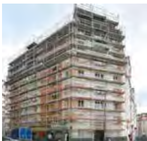
Scaffolding for cleaning the facade
