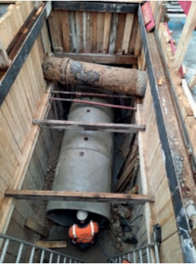
Placement of ovoid concrete elements
