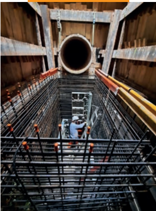
Installation of reinforcements
