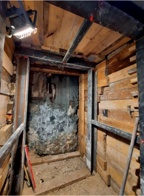
Gallery opening and support with wooden planches
