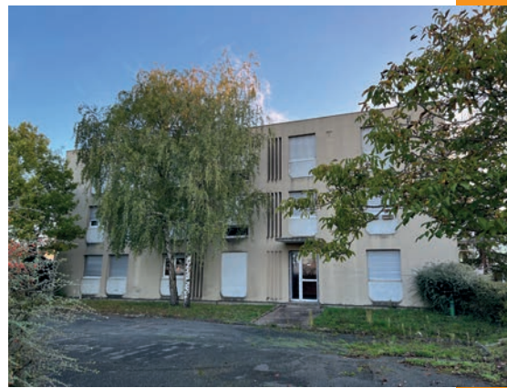
Building energy renovation project
