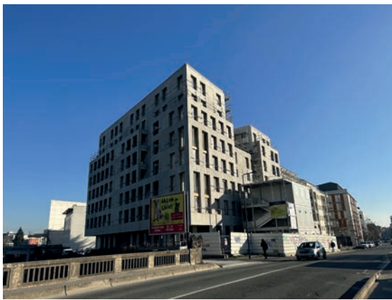
Construction project of 50 apartments.
