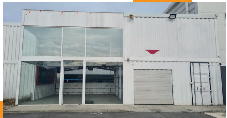
Photo of the current facade
