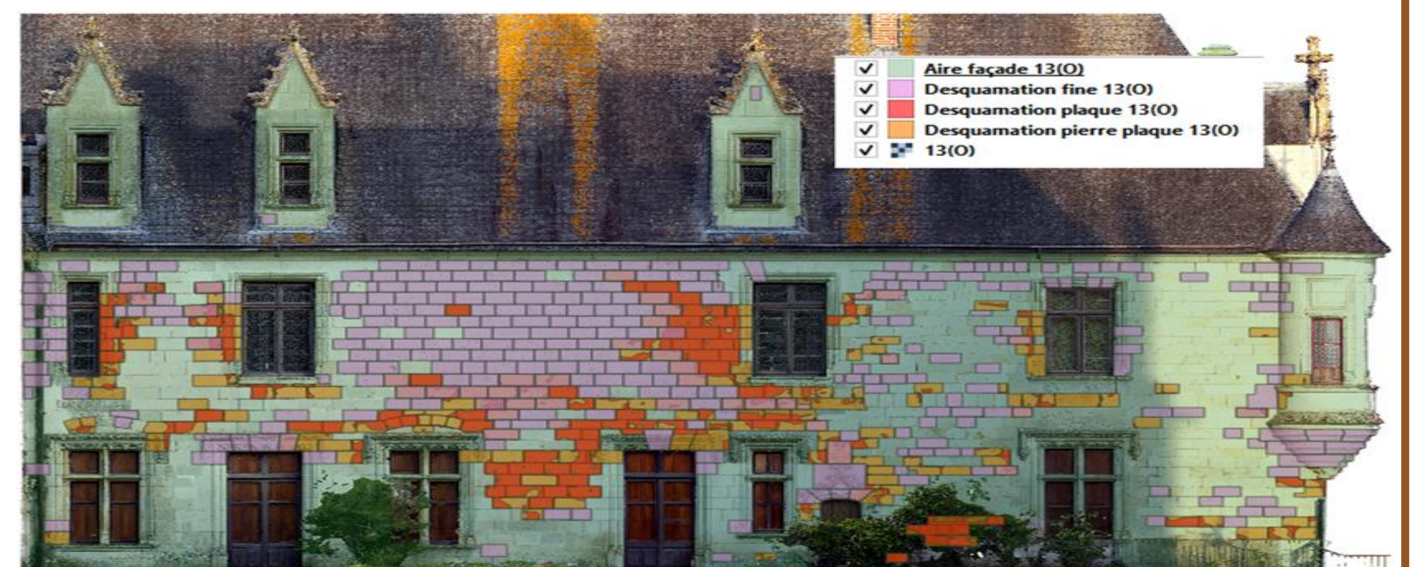
Orthoprojection of the façade No. 13 with degradation mapping (QGIS)
