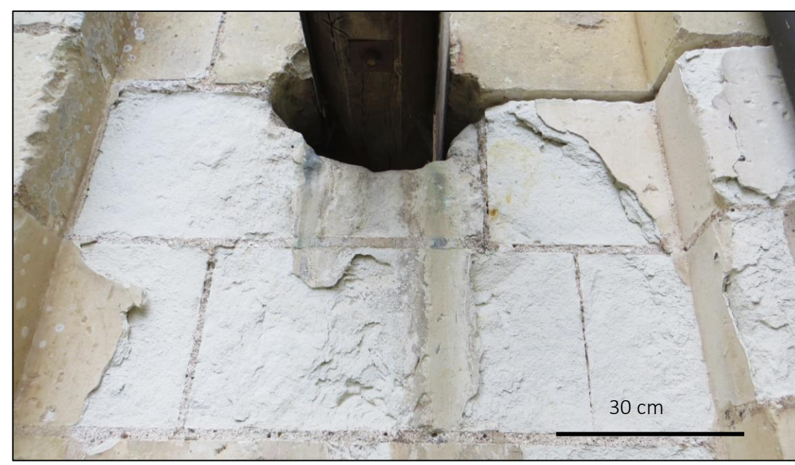
Example of spalling on tuffeau stone
