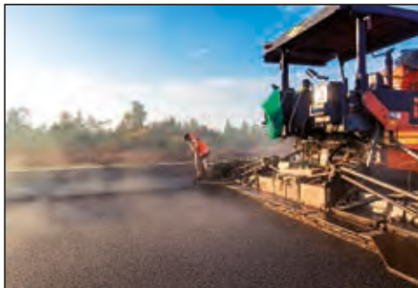
Application of hot asphalt
