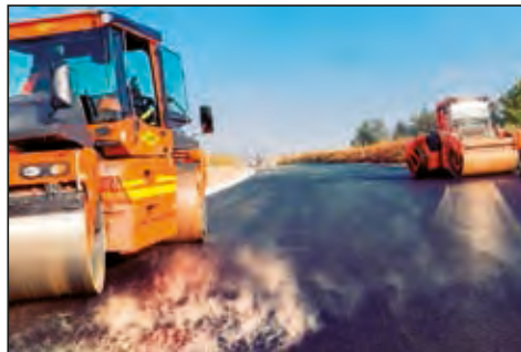
Compactors rolling the hot asphalt
