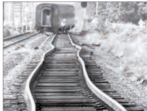
Thermal expansion of rails
