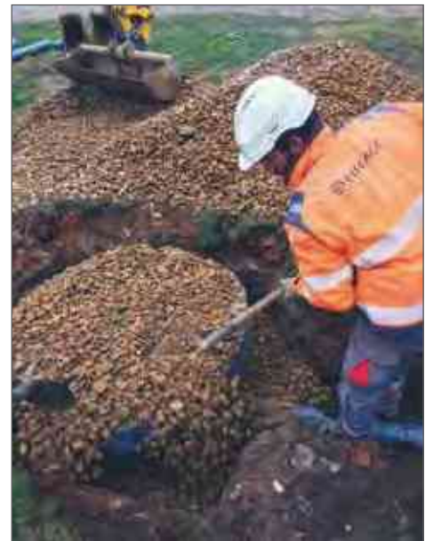
Installation of a sump
