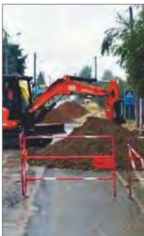
Construction of a trench for sanitation connection
