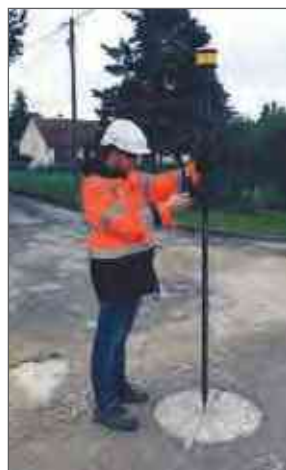
Use of the GPS rod to determine the altimetry
